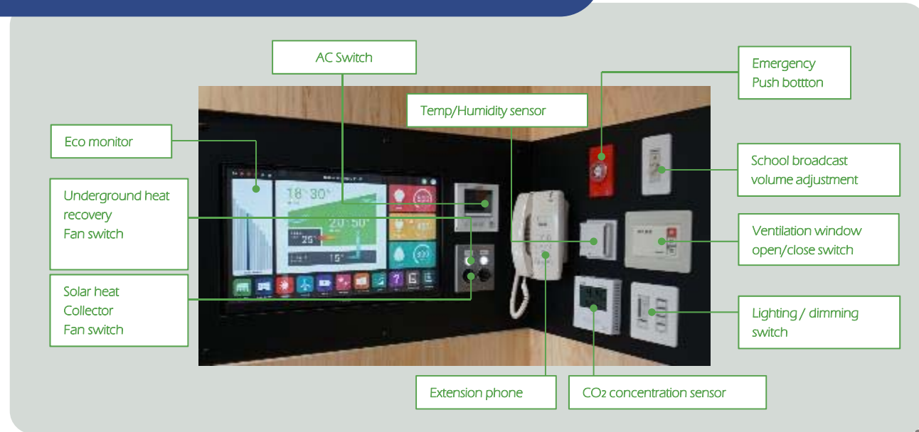
Eco monitor panel and switch
